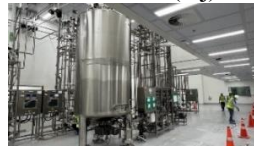
62 63 The Eat Just production facility being built in Singapore
